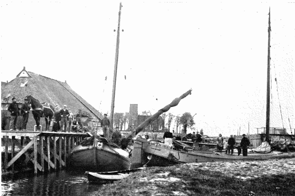
FIG. 2. Terpafgraving te Marsum (Fivelgo) in 1903. (Foto W.Pastoor).
